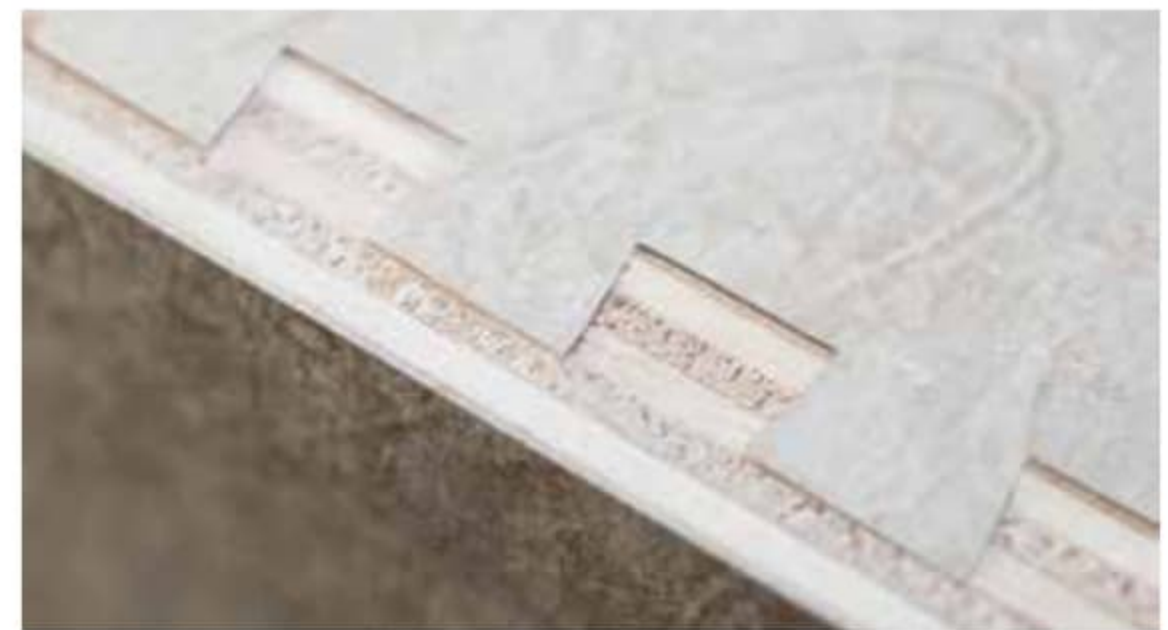
Residential dovetail drawer construction
